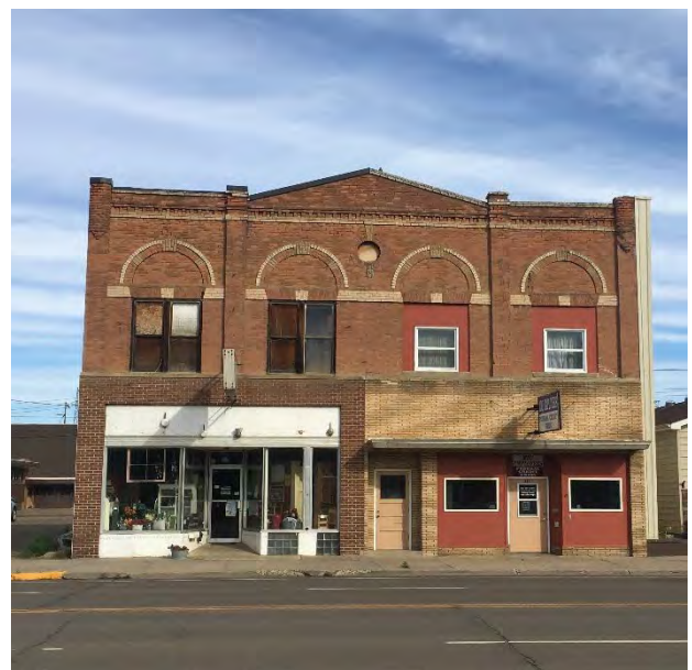
Image 12: When a facade is stabilized, the building can be prepared for renovation
